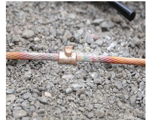
6. Remove weld and clean mold before making next connection.
