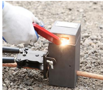
5. Ignite the starting powder with the Flint Ignitor.
