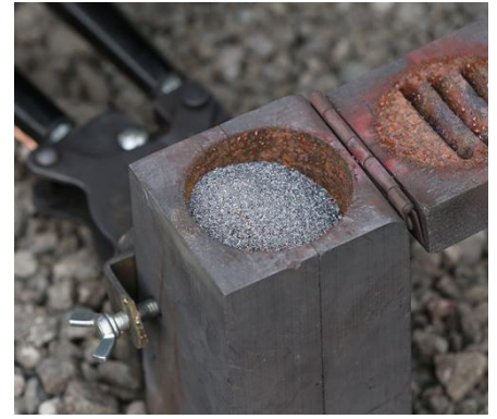
3. Dump weld powder into crucible.
